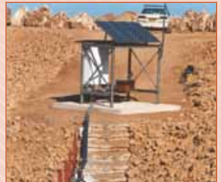
SOLAR POWERED HYDRAULIC FLOOD GATES
